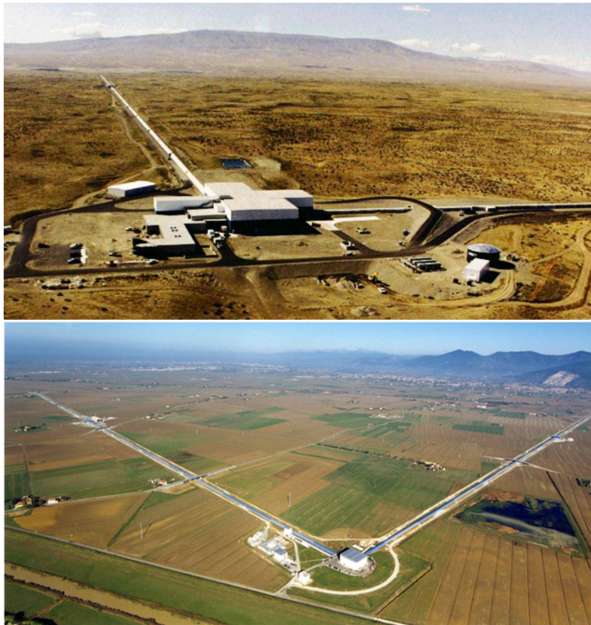
Figure 2.34. Top: Aerial view of the LIGO Hanford, Washington site. The vacuum enclosure at Hanford contains the 4 km interferometer. Photograph courtesy of LIGO/Caltech/MIT. Bottom: Aerial view of the Virgo detector, with 3 km arms, located near Pisa, Italy. Photograph courtesy of the European Gravitational Observatory.
