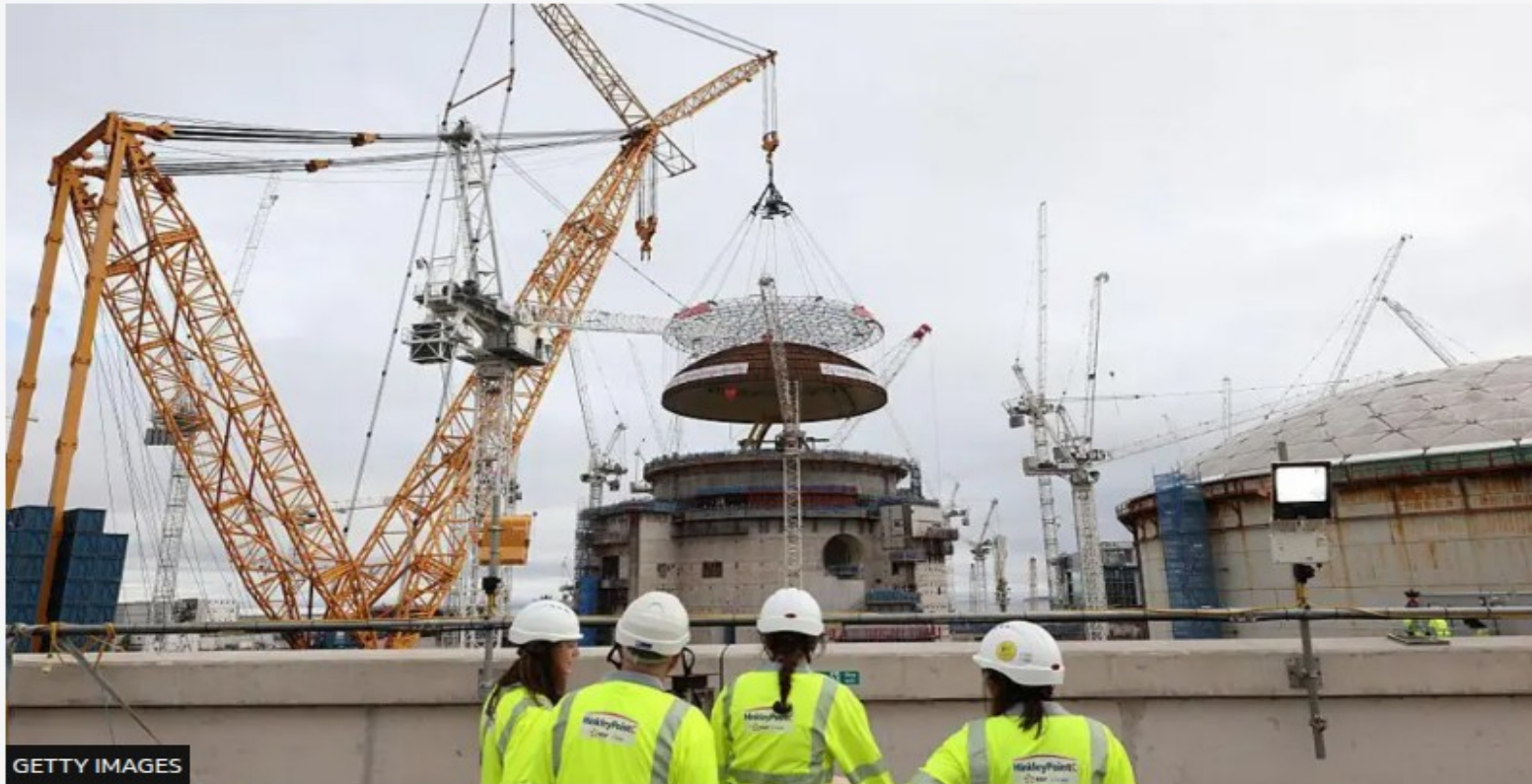
Hinkley Point C in Somerset is under construction
